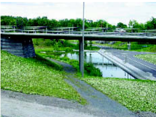
Dam i veianlegg (Fornebu).
