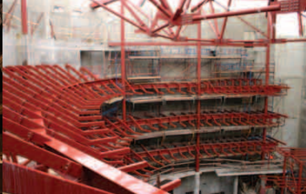
Steel constructions carry the balconies.
