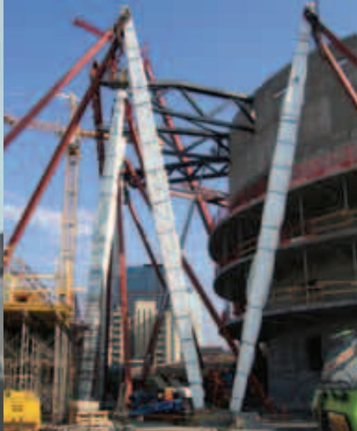
White, inclined concrete columns carry the weight of the roof in the foyer.
